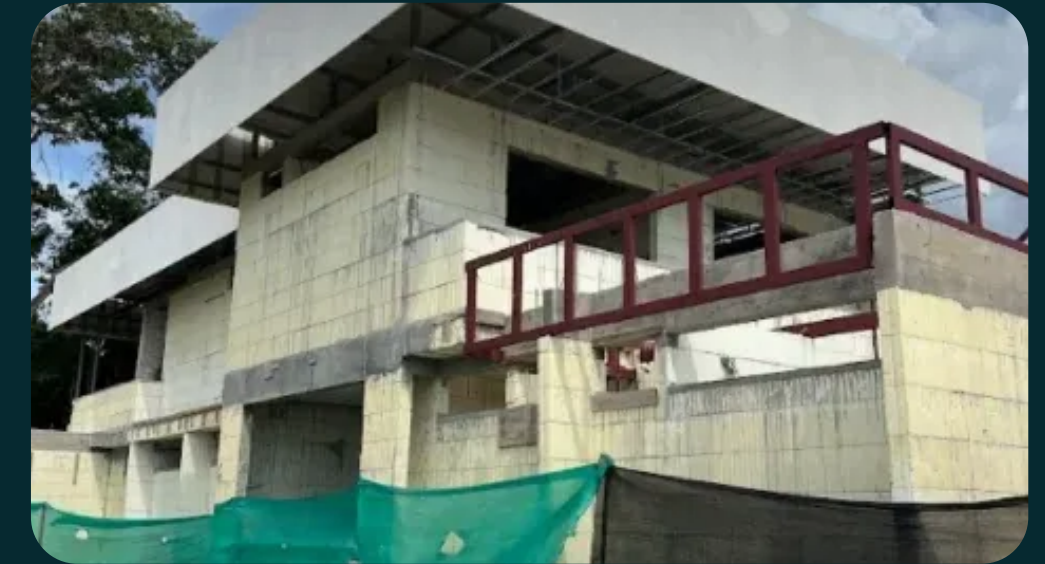
SANTA ANA URBANO HOUSE 94
