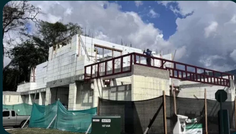
SANTA ANA URBANO HOUSE 92
